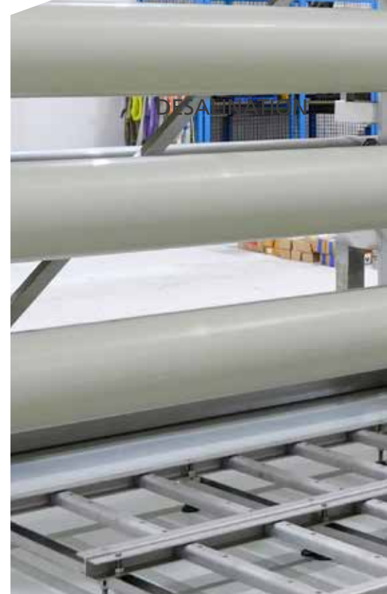
PE 100-RC SAND BED FREE INSTALLATION IN ALPINE TERRAIN
