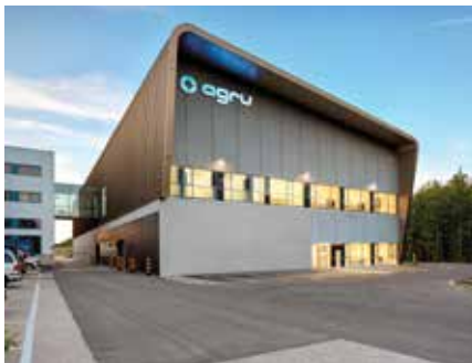
2019: EXTENSION OF PLANT 5
