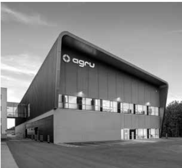
Figure B.1: New AGRU cleanroom plant.
