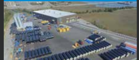
XXL PIPE PRODUCTION FACILITY CHARLESTON, SC/USA
