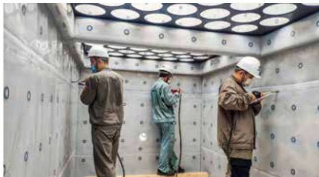
Bonding on steel
