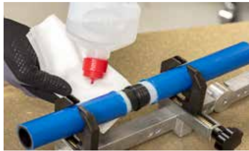
1. Cleaning of welded area
