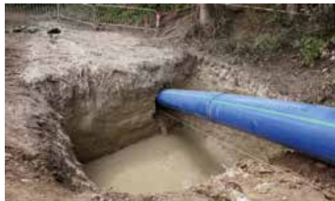
Horizontal Directional Drilling
